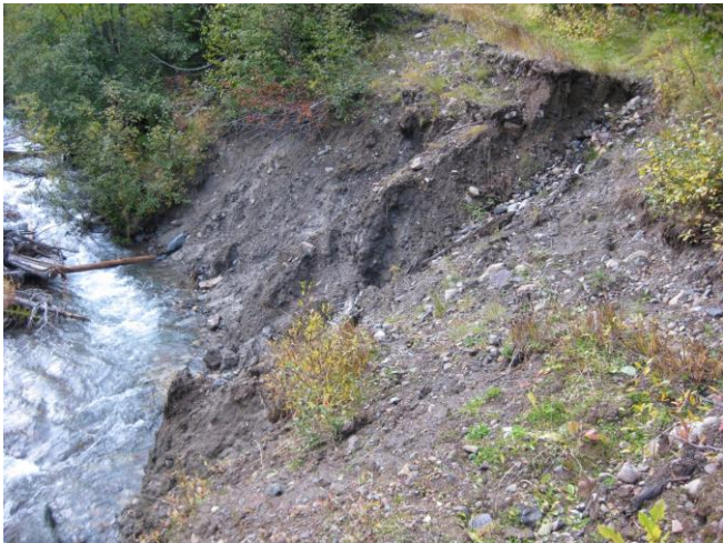
Figures 15 & 16. This is the site of the “Impassable Washout” as indicated in Figure 2. A large avalanche in 2007 caused the creek to change course, severely eroding the bank below the road to the point that there is no longer a road surface, just a slope directly down to the creek. Figure 16 was taken in 2008, there is now a 10m stretch of road that is just a slope.
