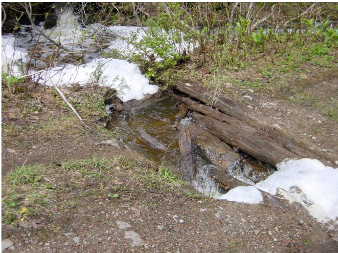
Figures 9 & 10. Failing wooden culverts between the trailhead and the Cronin Creek Crossing.
