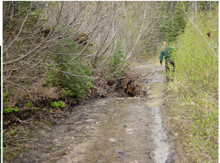
Figures 5 & 6. Many standing puddles of water along the entire stretch of road from the trailhead to the lower mine site, and a slope above the road slumping down onto the road about 1km before Cronin Creek (2006).
