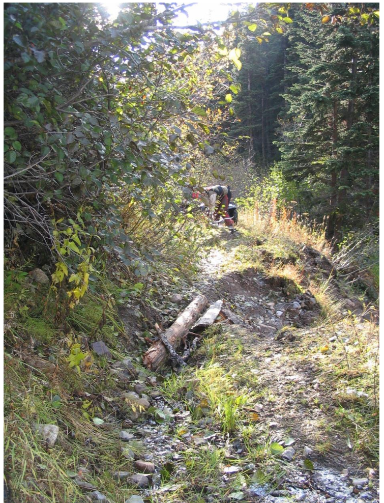
Figures 15 & 16. This is the site of the “Impassable Washout” as indicated in Figure 2. A large avalanche in 2007 caused the creek to change course, severely eroding the bank below the road to the point that there is no longer a road surface, just a slope directly down to the creek. Figure 16 was taken in 2008, there is now a 10m stretch of road that is just a slope.
