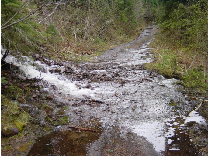
Figures 7 & 8. More examples of poor creek crossings. Figure 7 is about 500m before Cronin Creek. Figure 8 is the main crossing of Cronin Creek. Here, the original bridge collapsed and blocked the main flow, causing an entire new channel to form, making the crossing much more difficult and, for most of the year, dangerous.
