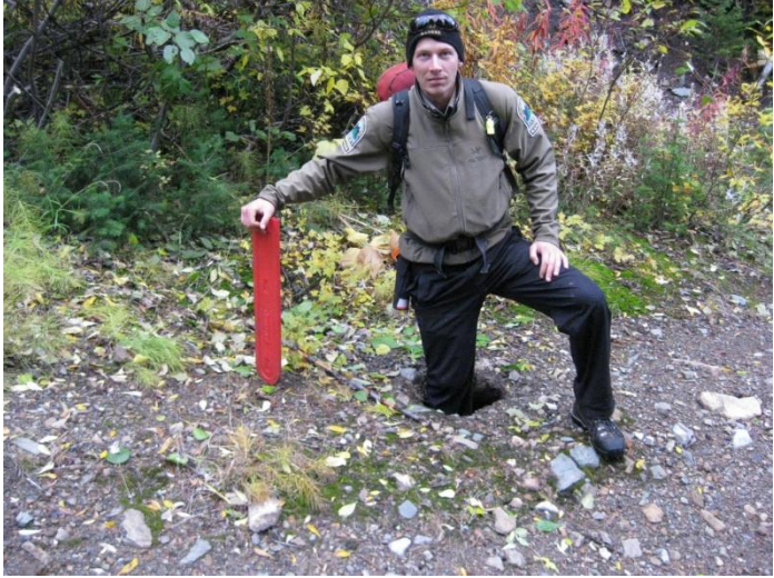
Figures 3 & 4. Holes forming in the road where wooden culverts are collapsing, and lack of cross ditching allowing creeks to flow down the road. Both taken above the lower mine site.
