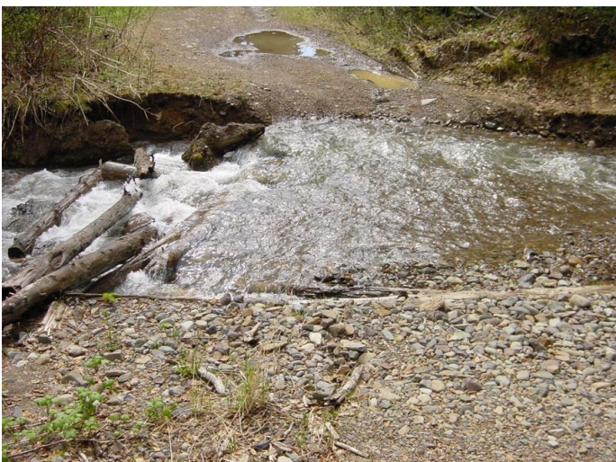
Figures 11 & 12. Failed bridge at a creek crossing about 3km from the trailhead. Figure 12 shows the cause of the "Large Gully Forming" as indicated in Figure 2. A 300m long gully has formed and grows annually as the water erodes it, taking the road surface with it.
