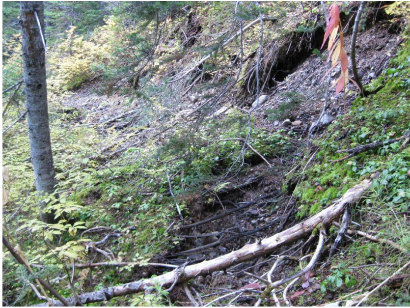
Figure 17. The entire slope above the “Impassable Washout” is also slumping.
