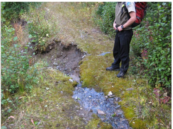
Figures 11 & 12. Failed bridge at a creek crossing about 3km from the trailhead. Figure 12 shows the cause of the "Large Gully Forming" as indicated in Figure 2. A 300m long gully has formed and grows annually as the water erodes it, taking the road surface with it.
