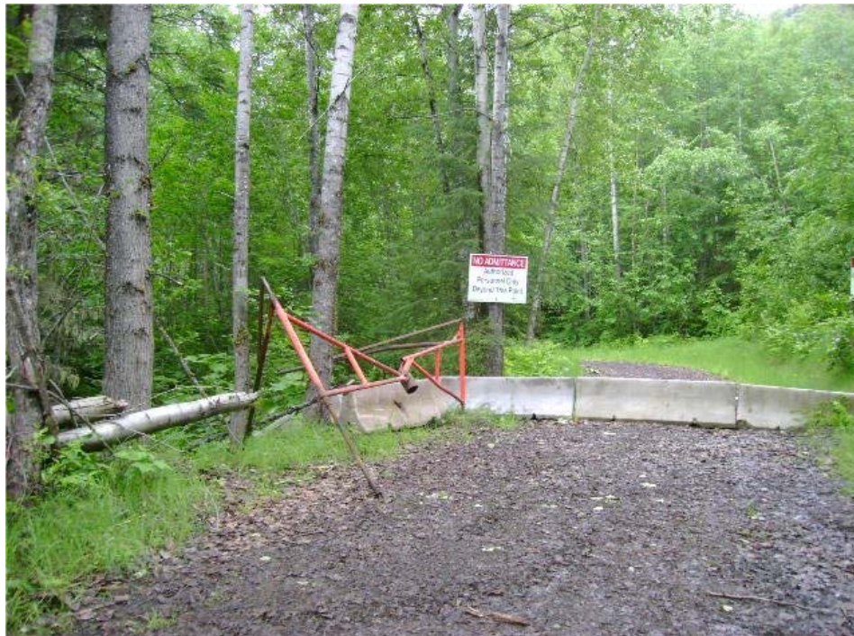
Figure 3: Gate removed. Upper barrier 30 June 2012.
